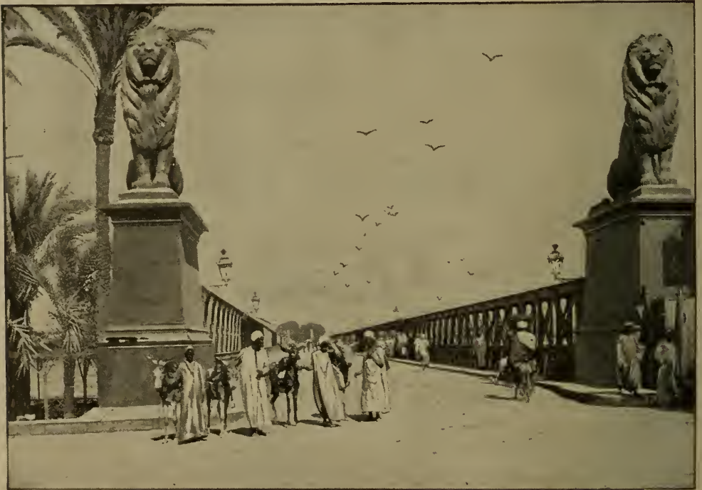
NILE BRIDGE AT CAIRO.
